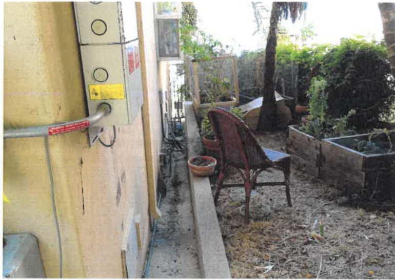
West side drainage channel and site landscaping looking south.
